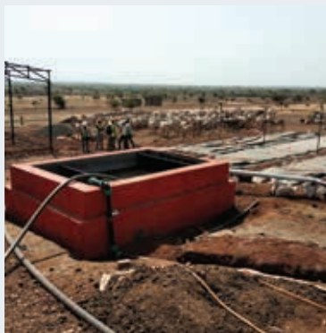
Community biogas plant under construction in Chipiya, Agar, Madhya Pradesh
